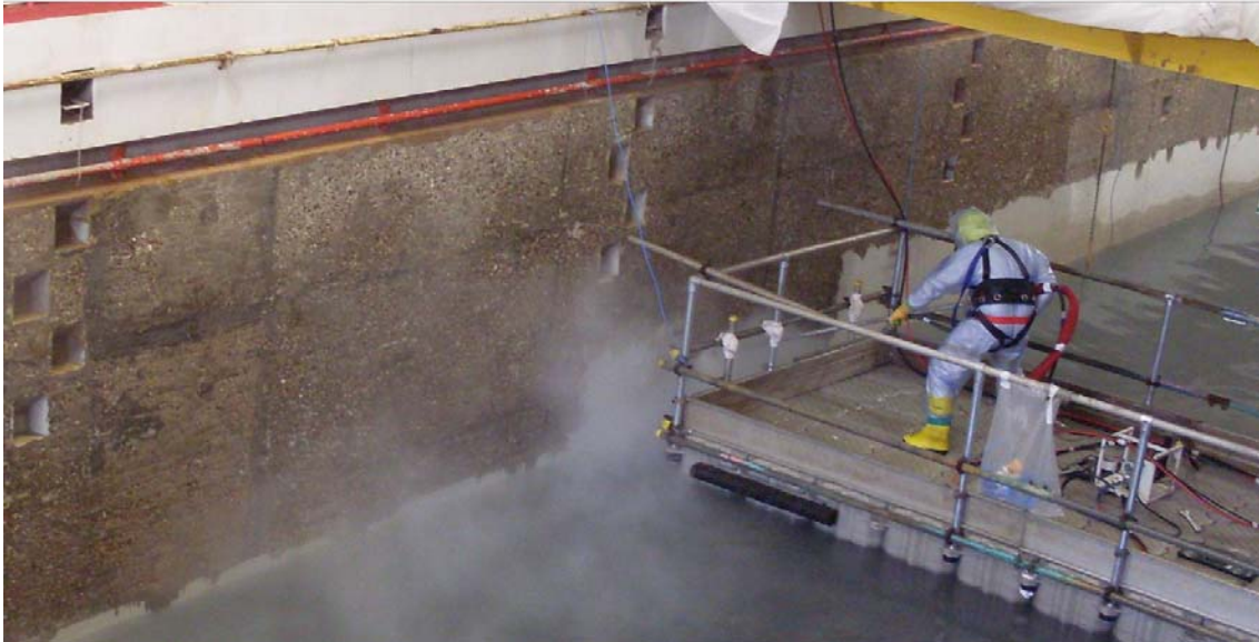
Figure 31.3-2 Decontamination of ponds at Bradwell using UHP water jet [Ref. 31-33]
