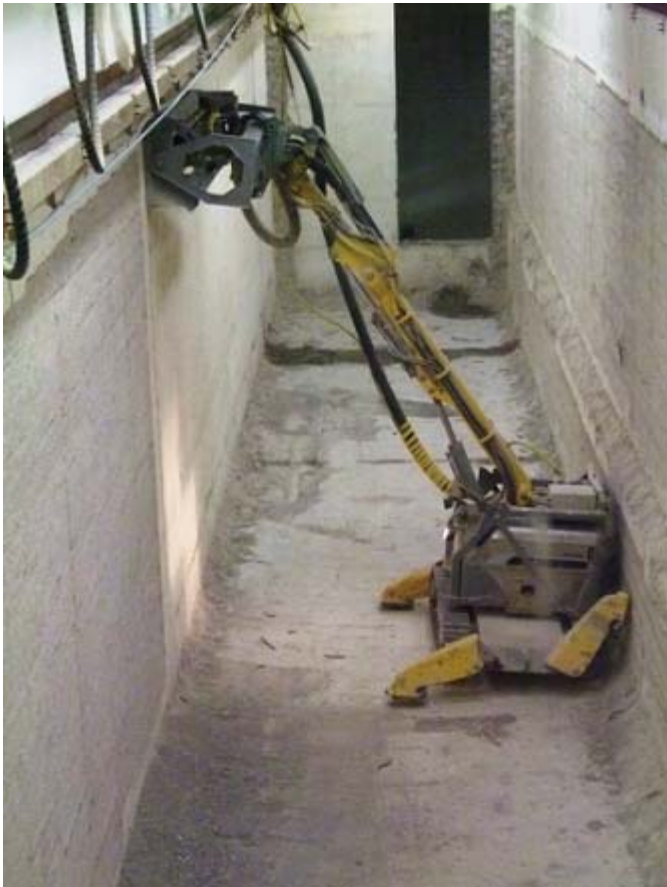
Figure 31.3-1 Scabbling pond walls at Trawsfynydd [Ref. 31-33]
